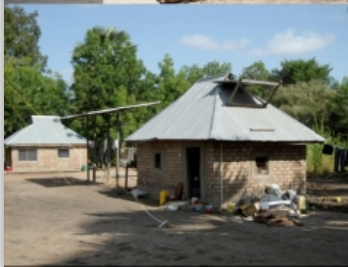
Clinic and school installation with hands-on training
