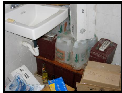
Figure 5: Old batteries stored in the bathroom of a health facility. Battery recycling is economical and environmentally sound.
