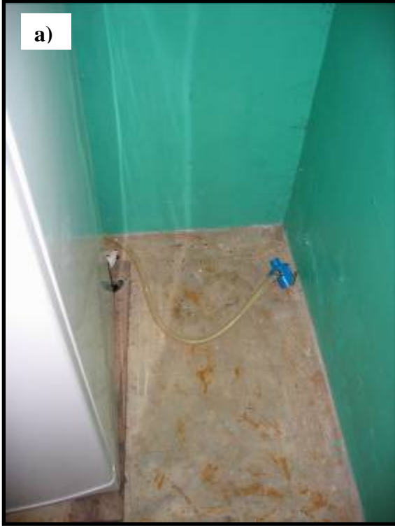
Figure 3: a) CDC provided blood lab refrigerator not connected to gas or electric power b) gasket on refrigerator faulty, c) contents of refrigerator at room temperature, d) temperature log out of date, and e) blood bank refrigerator not in use because of insufficient power.
