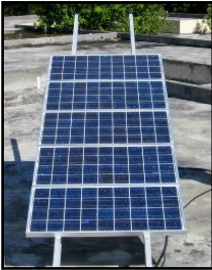
Figure 1: WHO installed solar powered vaccine refrigerator has worked well for two years. A smaller solar system has worked for 6 years powering the radio.
