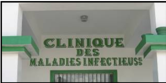
Figure 3: New buildings and equipment, such as the PEPFAR supported infectious disease building, have more than doubled the hospital's electrical load in the past four years with no associated upgrade of the internal wiring and circuitry.
