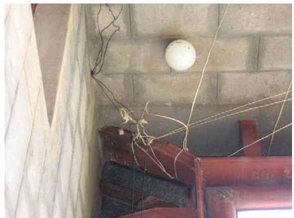
Inadequately sized and hung wire connecting buildings at a health center.
