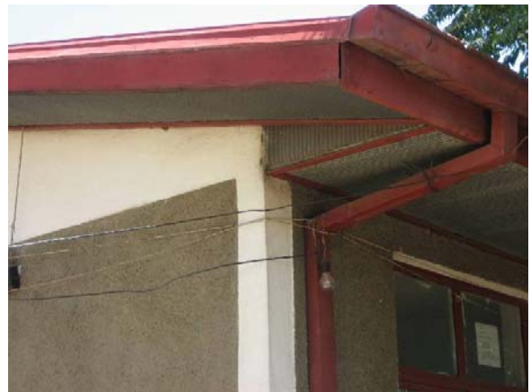
Inadequately sized and hung wire connecting buildings at a health center.
