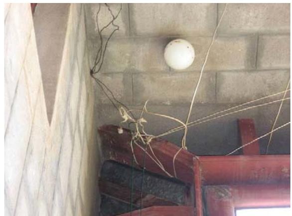
equipment has been added, or buildings have been added, the wiring has been installed at improper sizes, and without concern for adequate fuses, circuit breakers, or grounding.
