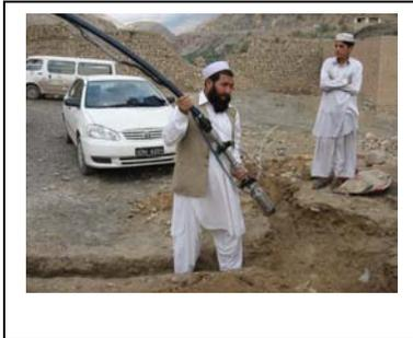
It was Saturday when we were ready to make the down-hole assemblies for the piping and the wiring in the wells. This included assembling all of the 1.25" piping along with the safety cable, the power cable, and low water probe cable into
