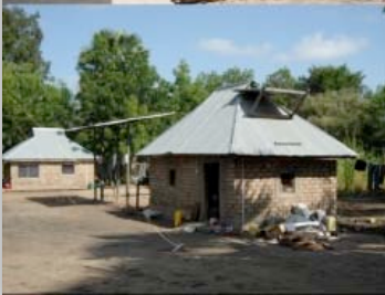
Clinic and school installation with hands-on training
