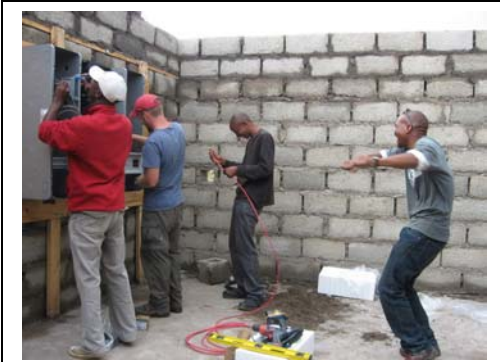
We're Almost done (Who needs a roof?)
