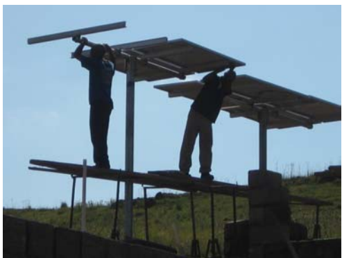
Installing panels on the poles.
