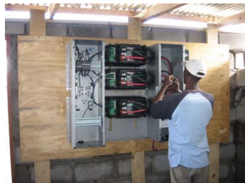
Wiring up the Inverters.
