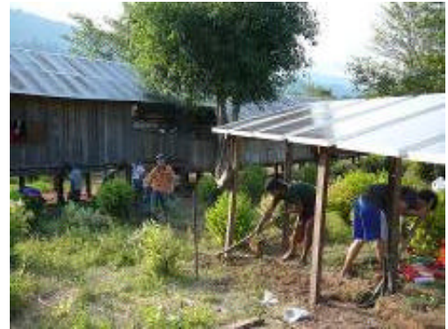
Medics work on the solar panel structure and wiring
