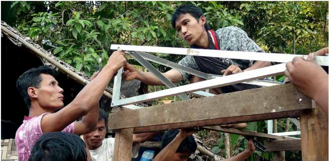
THAI MEDICS MOUNT ALUMINUM PANEL SUPPORTS ON A WOOD RACK IN ORDER TO INSTALL SOLAR PANELS AT A REFUGEE HOSPITAL.
