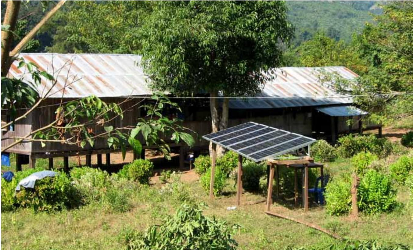
THE COMPLETED EQUIPMENT RACK OUTSIDE OF THE REFUGEE HOSPITAL PROVIDES SOLAR ENERGY TO POWER OUTLETS FOR MINOR SURGERY, LABORATORY MICROSCOPES, COMPUTERS, VACCINE REFRIGERATORS AND LIGHTS. PHOTO | COURTESY OF WALT RATTERMAN
