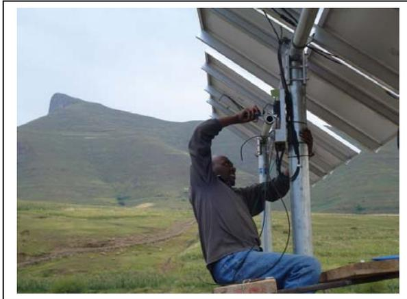
Once we arrived at a given site, our work was to (a) oversee the completion of the electrical buildings with special attention to the details needed to accommodate the energy equipment, (b) help with the installation of the galvanized steel poles for the mounting of the solar arrays, and (c) proceeding with the installation of the solar panels, inverters, batteries and all of the auxiliary equipment.
