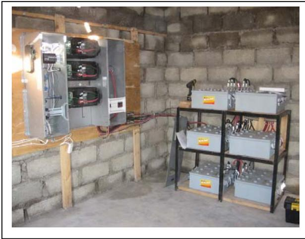
With this in mind, the Phase 1 systems for each site include all of the basics of a solar / diesel hybrid system, including the inverter equipment, charge controllers, batteries, solar panels, and a connection to the generators being delivered to the sites under other programs. The quantity of the solar panels and batteries are designed, in this initial phase for the needs of the VSAT and communications equipment along with other limited loads.
